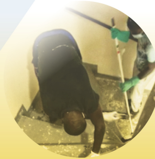
Phase 2 / cleaning 8 floors
